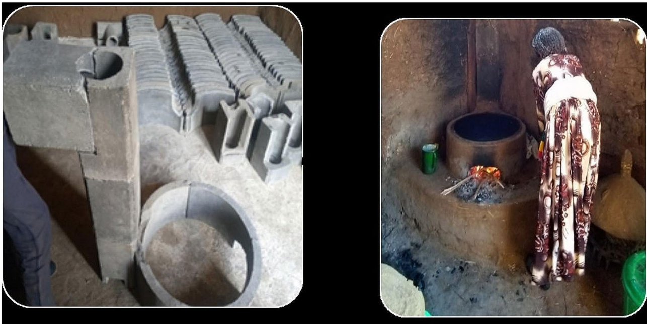
Fig. 1 Chimney fitted Mirt stove technology in the stock before installation and after the installation
